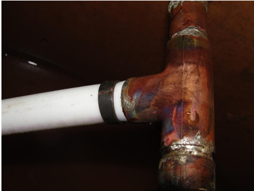
Tee installed and PEX attached
