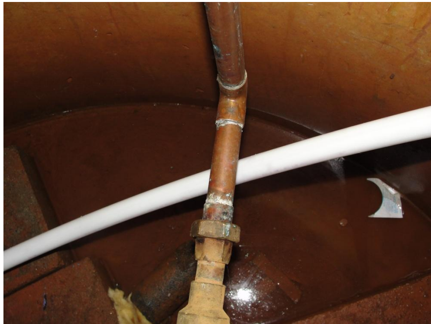
Gauging location of tee and length of PEX required
