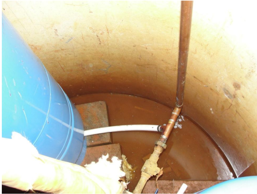
Pressure tank fully installed
