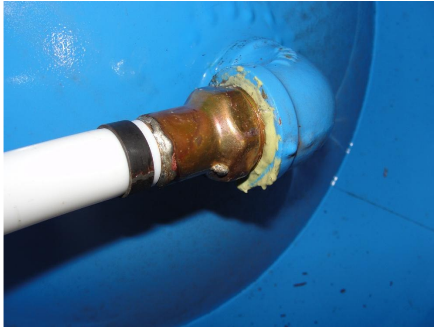
Installing PEX adapter onto tank
